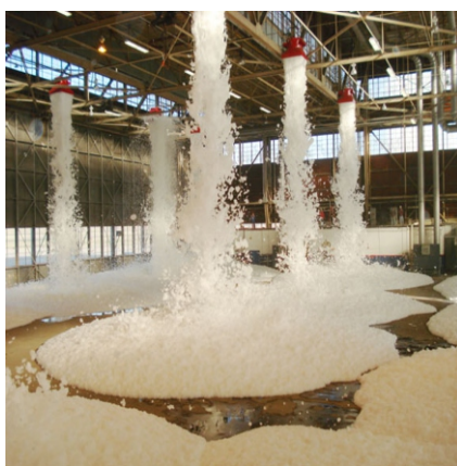
Foam System Discharge
