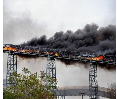
Conveyor Belt Fire
