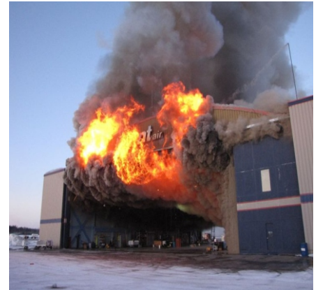
Aircraft Hangar Fire
